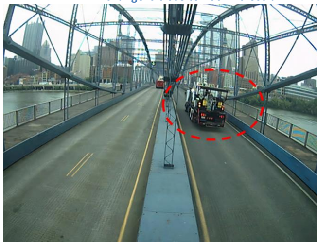
Figure 4: The photo of the truck captured by the camera on a truss bridge. The time tag from the camera is 08/20/21 at 09:22:40am, which matches the time of the high strain event.
