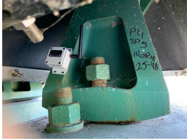
Resensys Wireless Tilt/ Inclination SenSpot sensors on bridge bearings to assess bearings functionality
