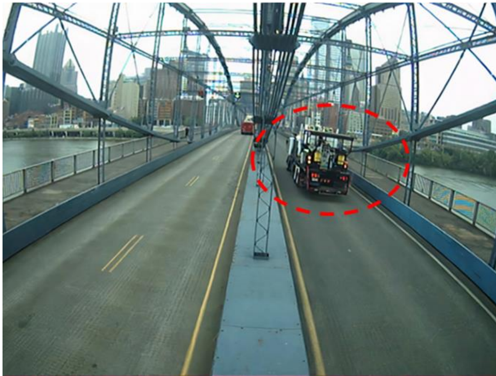
The photo of the truck captured by the camera on a truss bridge. The time tag from the camera is 08/20/21at 09:22:40am, which matches the time of the high strain event.
