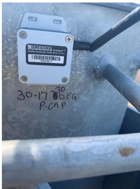
Wireless Accelerometer (3D Vibration) SenSpot™ installed at a turbine structure
