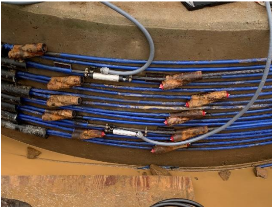
Wireless Displacement gauge (Crack meter) SenSpot™ installed outside surface of the turbine base to monitor potential crack at outside surface of the turbine
